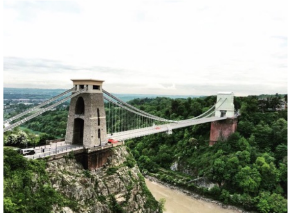
Clifton Suspension Bridge( Bristol知名地標)
